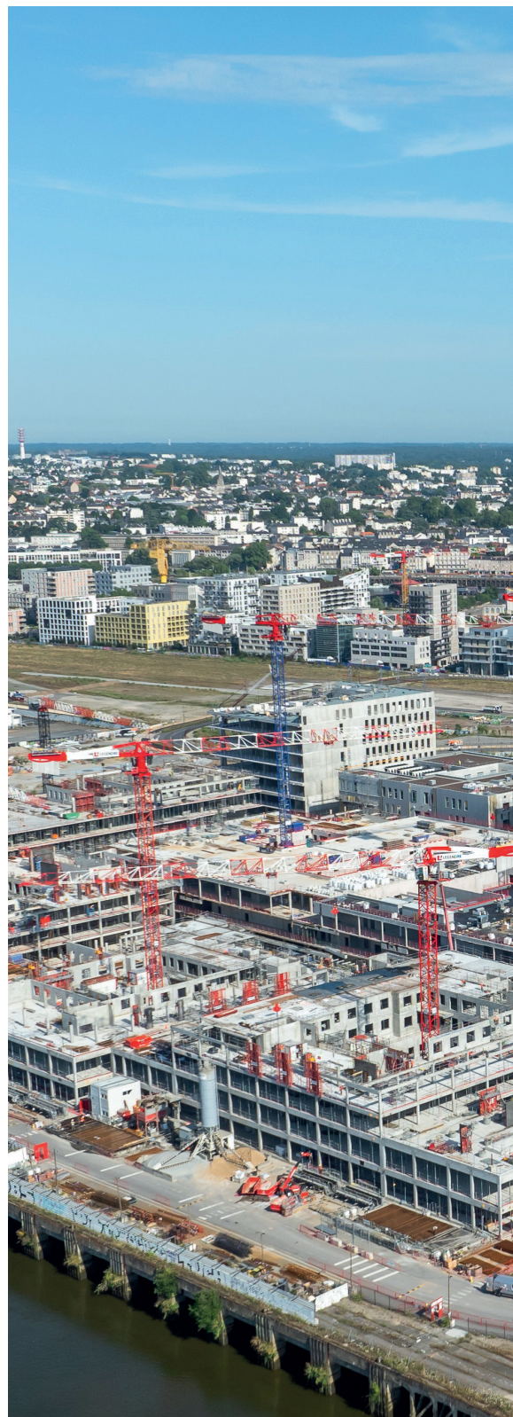
The new Nantes University hospital in France uses two types of Exegy low-carbon concrete in 7 of its 13 buildings.
