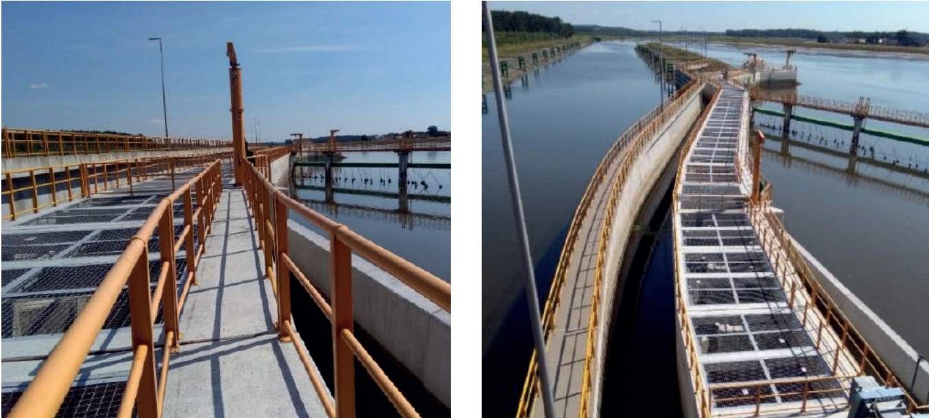
Figure 12: Fish ladder at the Malczyce barrage presented as a good example. However, this is not an action taken to achieve good water status. It is a measure to mitigate the negative impact of new hydro-technical investment – the obligation to implement it results from article 4.7 of the Directive (“all practical steps have been taken to limit the adverse effects on the status of the water body”), not from article 11. No other mitigating measures in the environmental decision enabling the implementation of this construction have been implemented. Source: International Odra draft RBMP, page 100.
