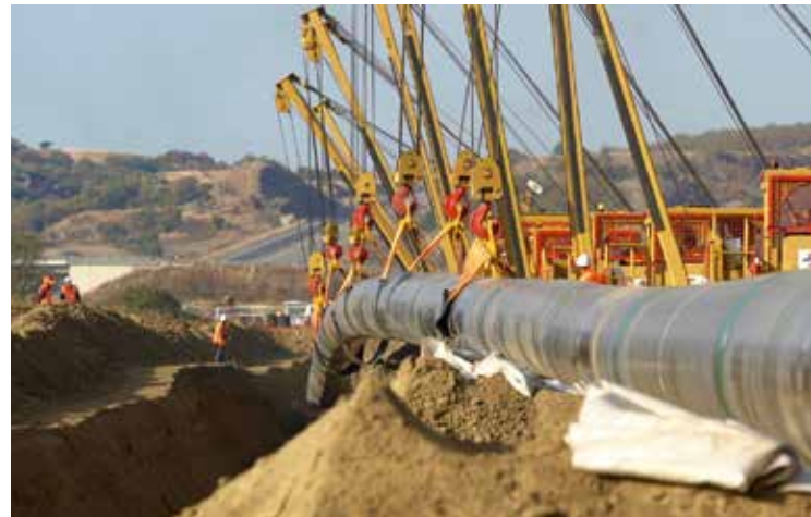
Works are ongoing to build the controversial Trans-Adriatic Pipeline, which will transport gas from the Caspian Sea to the Mediterranean at a time when more investments in renewable grids are needed. Source: TAP-AG
