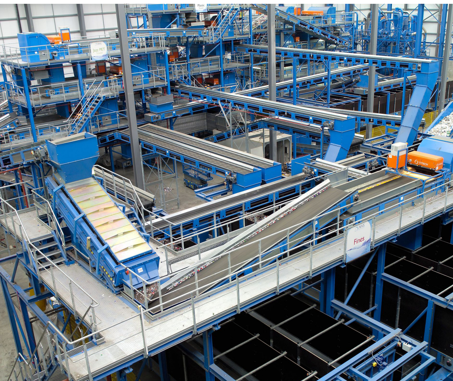
ECO Plastics reprocessing plant in the UK - the world's largest plastic bottle reprocessing facility.
